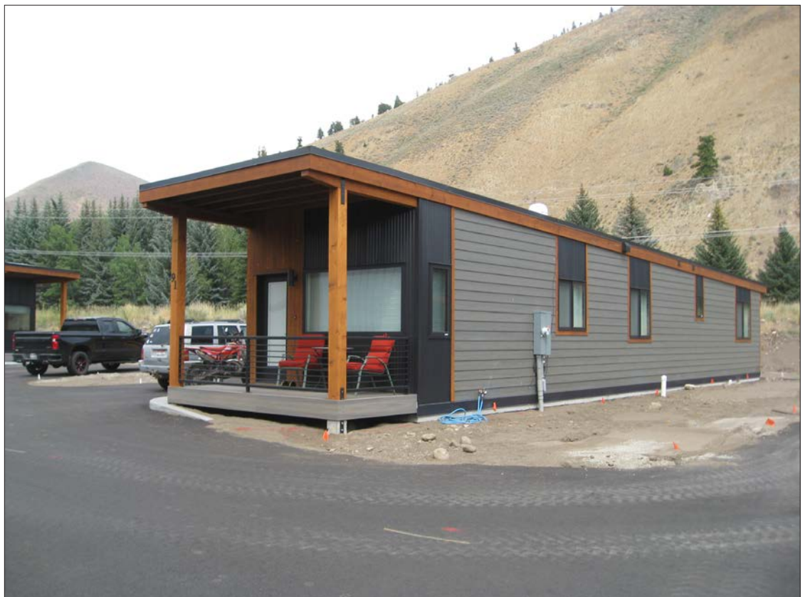
One of the eight new prefabricated housing units at the Greenhorn fire station. Photo credit: WRW Staff
