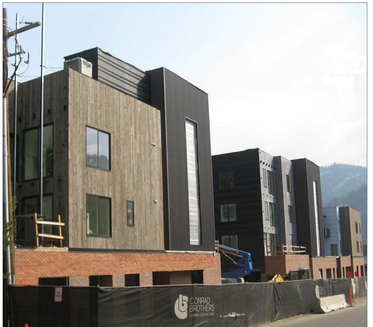
Bluebird housing project under construction in Ketchum. Photo credit: WRW Staff
