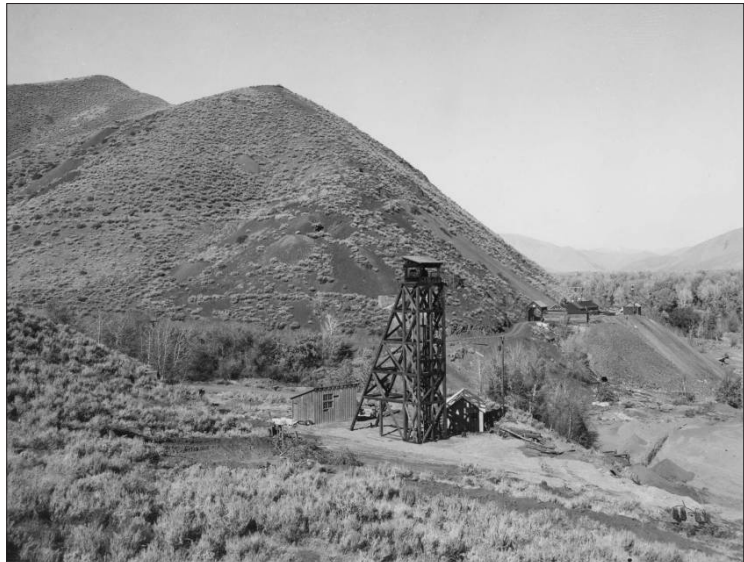
Headframe of the Queen of the Hills Mine near Bellevue, Blaine County, Idaho. The Silver Star Queen Mine is in the background. Mine buildings at the Silver Queen are erected on the waste dump above the forested valley floor. Photo credit: Idaho State Historical Society
